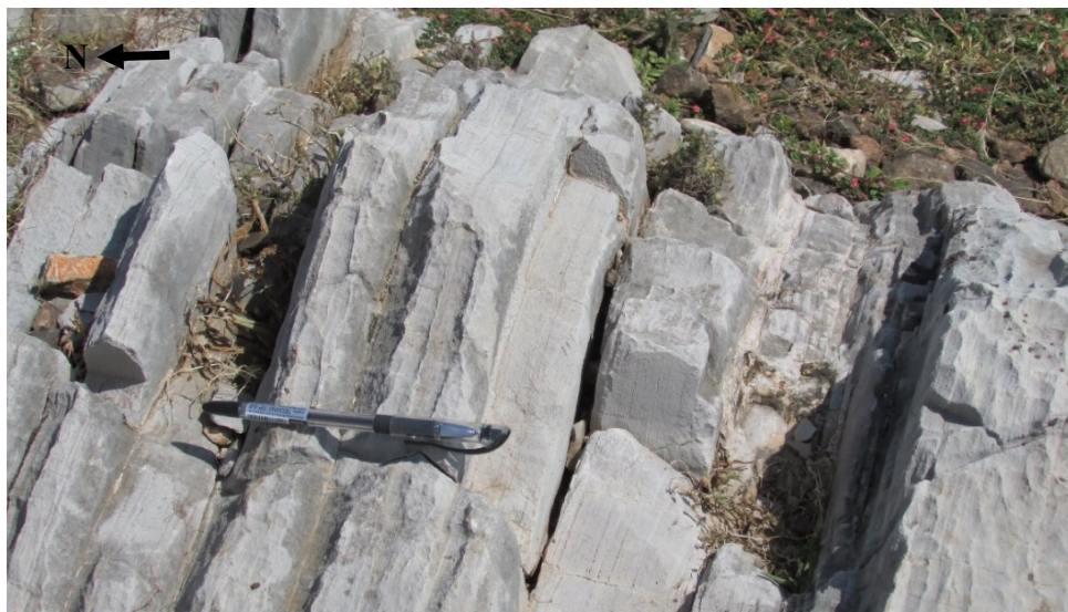
Fig 4: Steeply dipping limestones reflect surface expression of the Kurlagere-Gogi-Gundanahalli fault. Location: West of Gogi.
